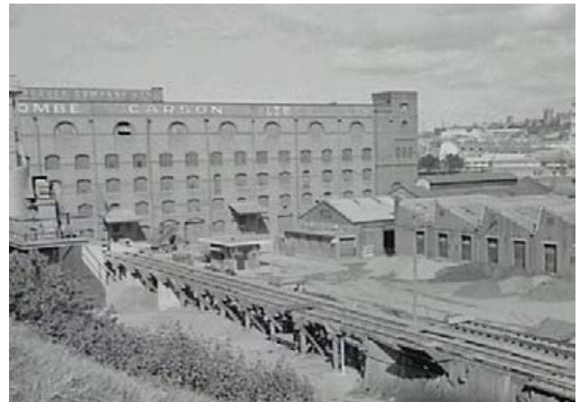
Wincombe Carson Ltd and Wentworth Park in background, 27/07/1962 Source: Sydney City Archives, NSCA CRS 48/2655
