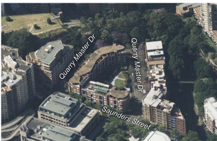
Figure 74 – oblique aerial of 26-38 Saunders Street
