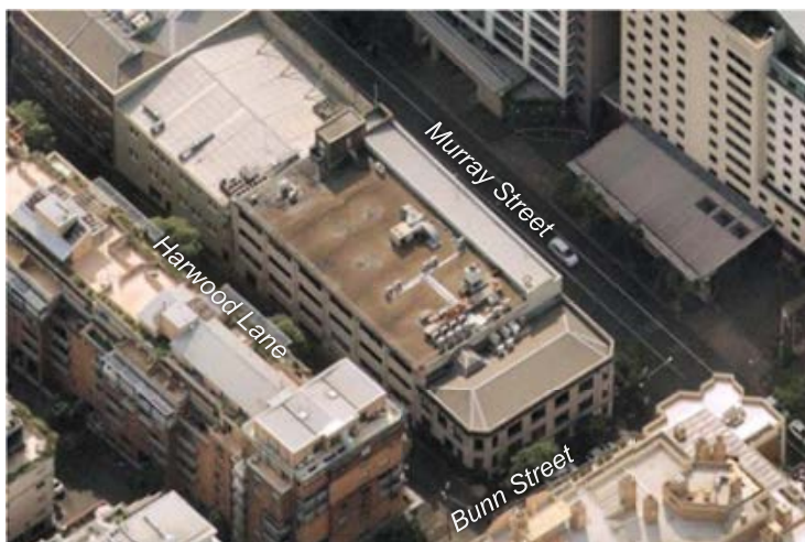
Figure 56 – oblique aerial of 55-65 Murray Street
