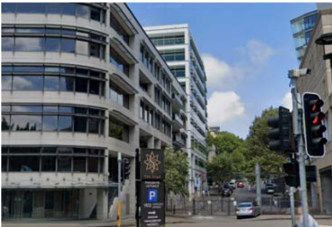
Existing – from Pirrama Road
